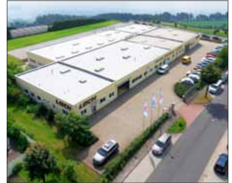
Plant in Lichtenau near Chemnitz, Germany
