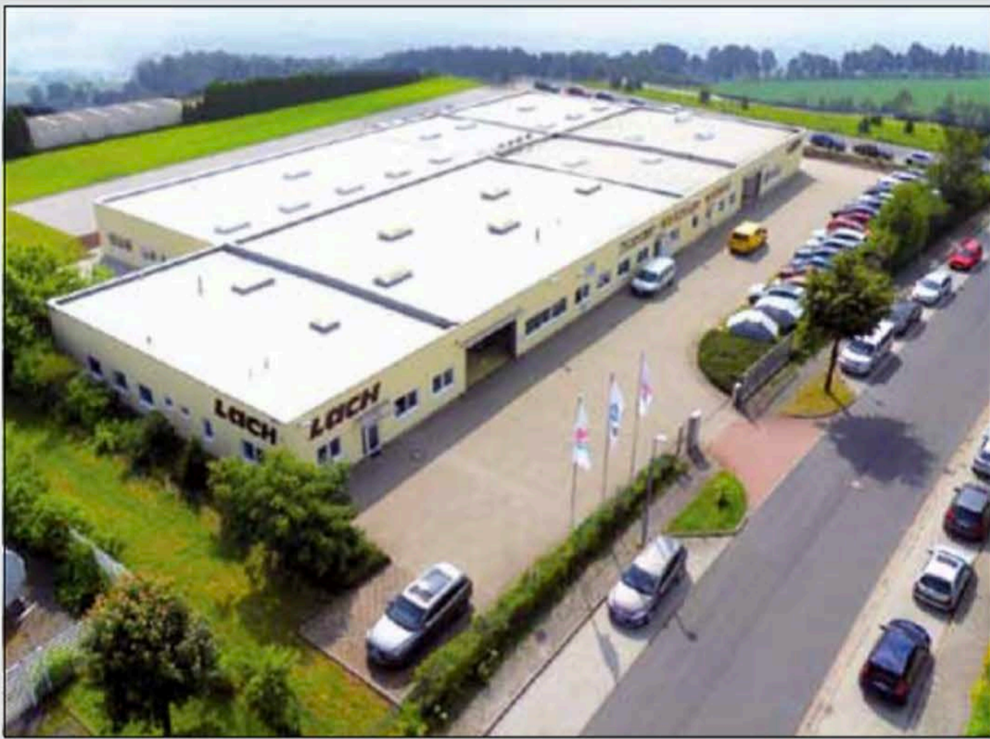
LACH DIAMANT facility in Saxony, today after 3 rd building section.
